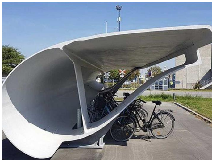
Figure 6.4: Section of a wind turbine blade repurposed as a bike shelter in Denmark
